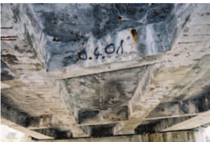
Concrete deterioration.
